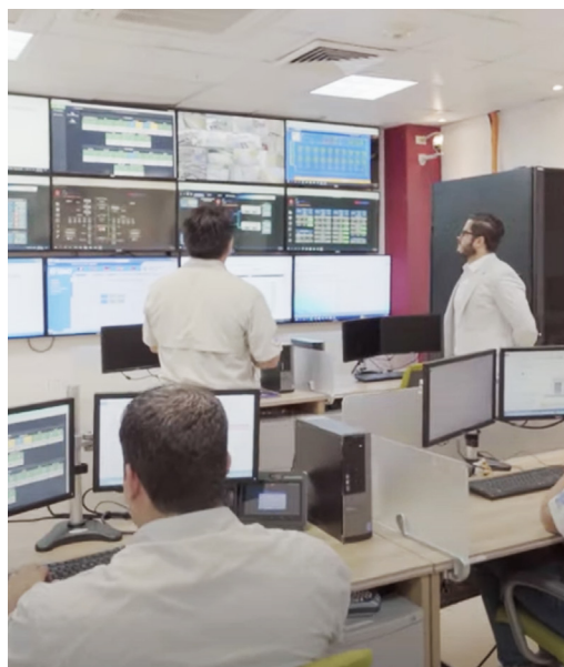
Our Panama City data center.
