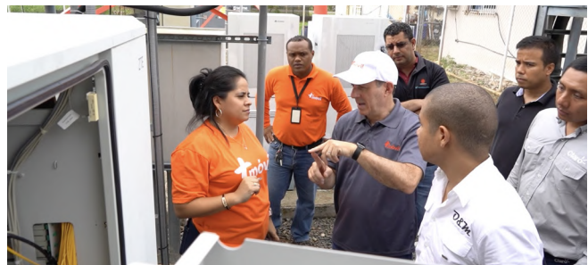
Tour of facilities by our leaders and team of technicians in Panama.
