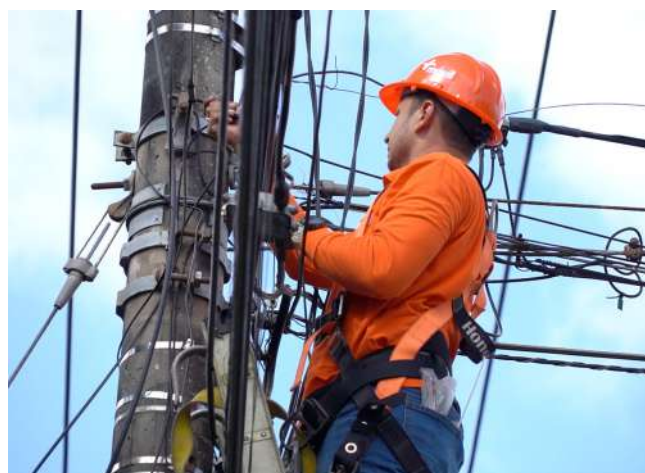
Our +Móvil and Liberty Costa Rica technician maintaining phone and broadband connection in Panama and Costa Rica.
